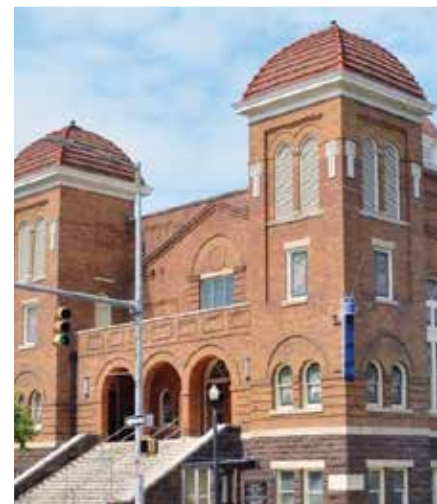
SIXTEENTH STREET BAPTIST CHURCH Birmingham, Alabama
